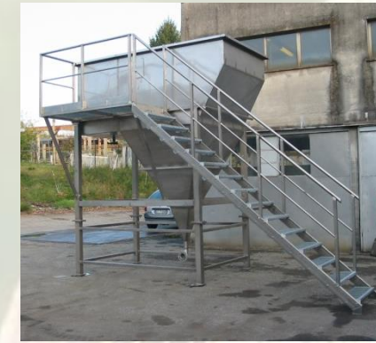
Additional tank for different treatments (double control of pH, chromates reduction, coagulation, etc).
